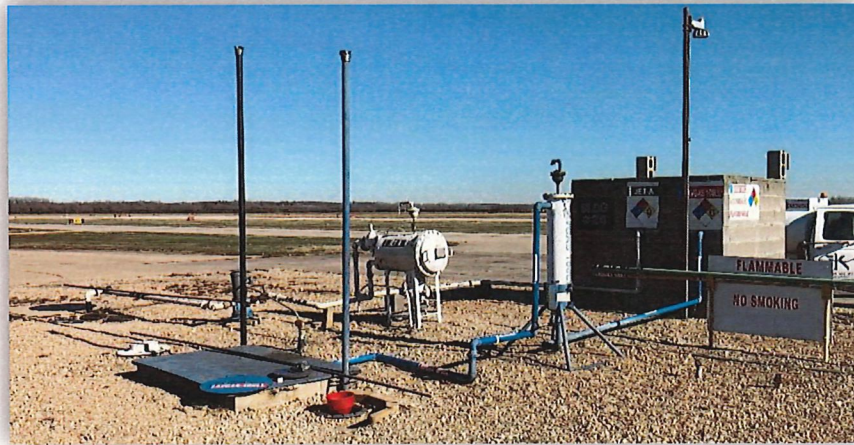
Existing Fuel Facility
